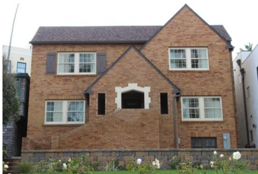
Historic Restoration of the Swansea Apartments; Hotel Expansion. Circa: 2019
